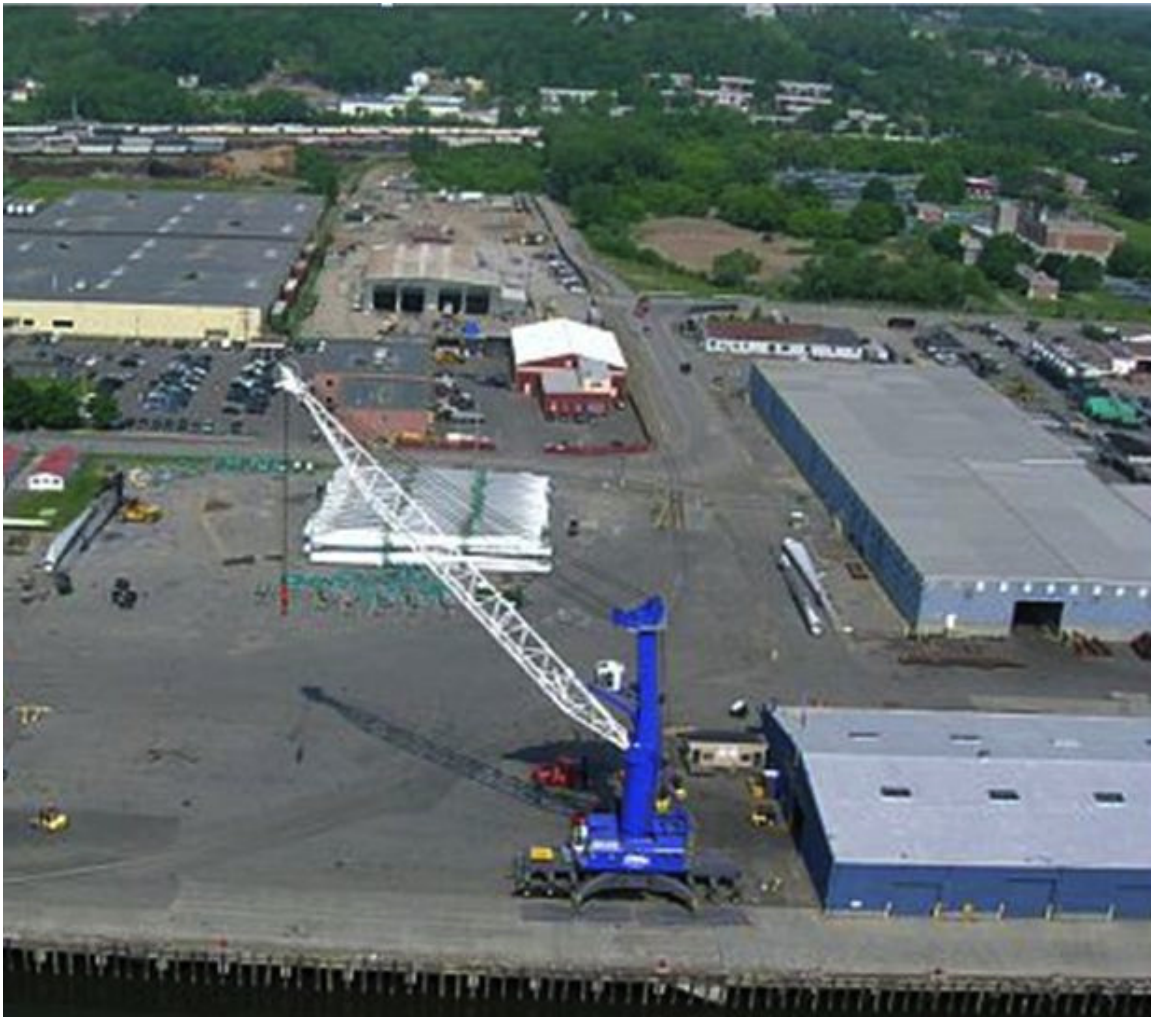
Figure 8: Container crane at Port of Albany
