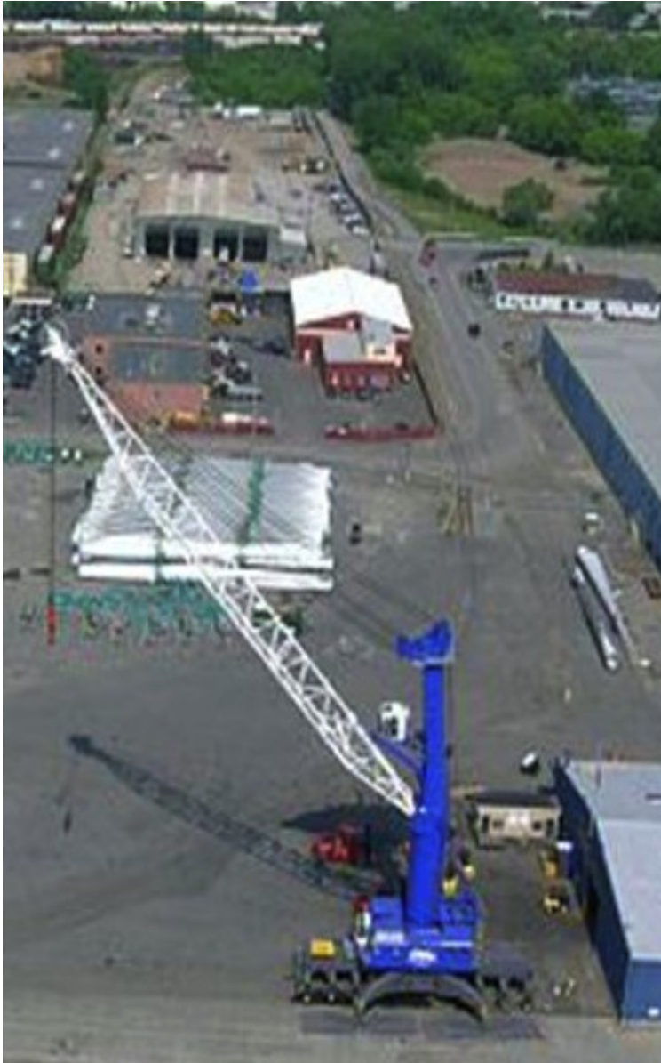
Figure 4: Container crane at the Port of Albany
