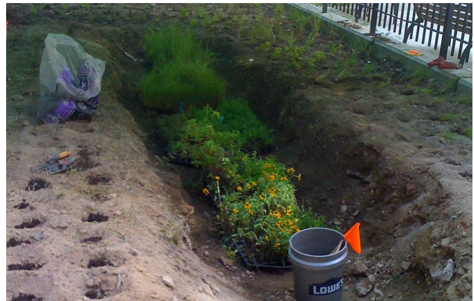
Above: the site was infested with Mugworts nearly five feet high and strewn with trash. Below: after weeding, a ditch was dug out for a wetland. Holes on the left were dug with a jackhammer. Because of the location of the site, removal of the top layer of soils was not possible. Far left: the site was planted with all native species. Inside the ditch, wetland species were planted.
