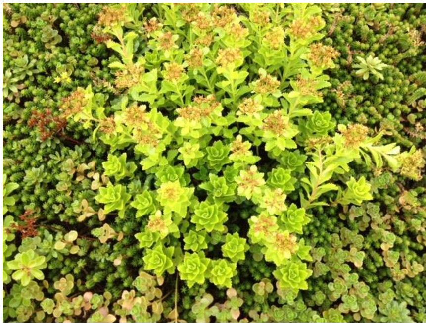
Sedum on the greenroof at Logan Gardens. A Spruce sapling was found growing on this roof!
