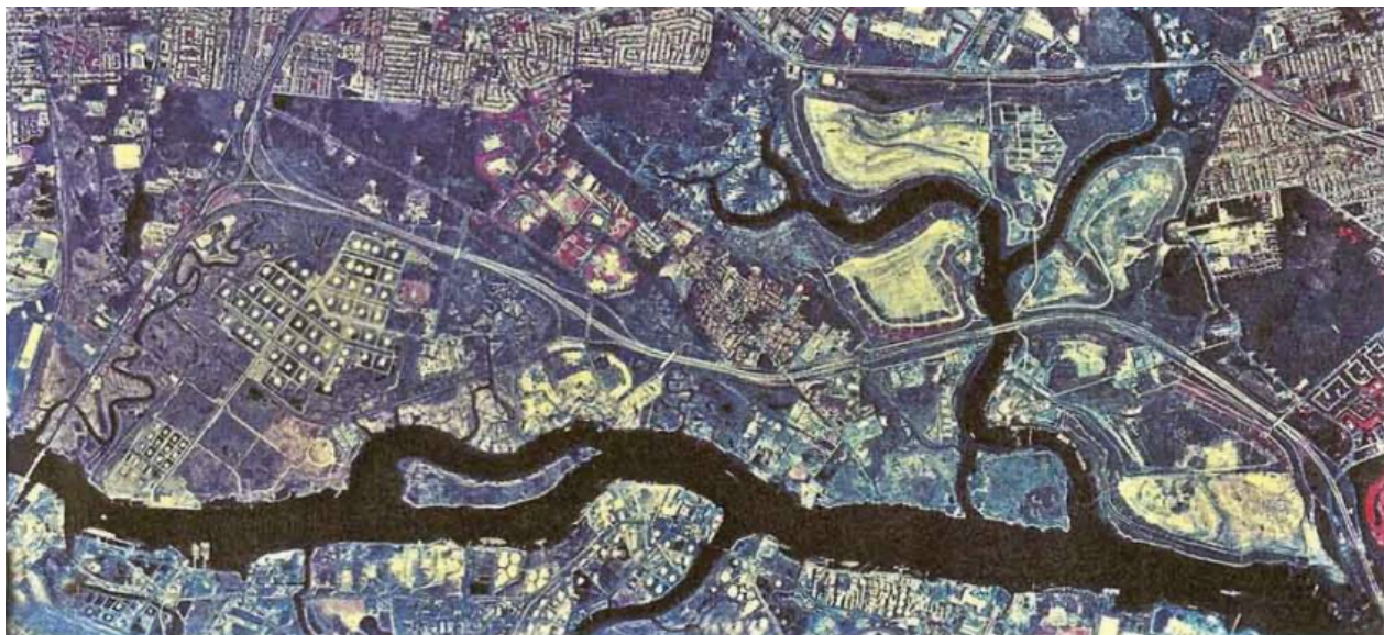
Tidal wetlands of the study area, along the Arthur Kill, including an oil tank facility on former wetlands. Source: p. 14 Tiner, R. (2000).
