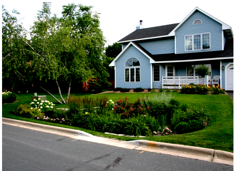
Rain garden. Source: The US Environmental Protection Agency.
