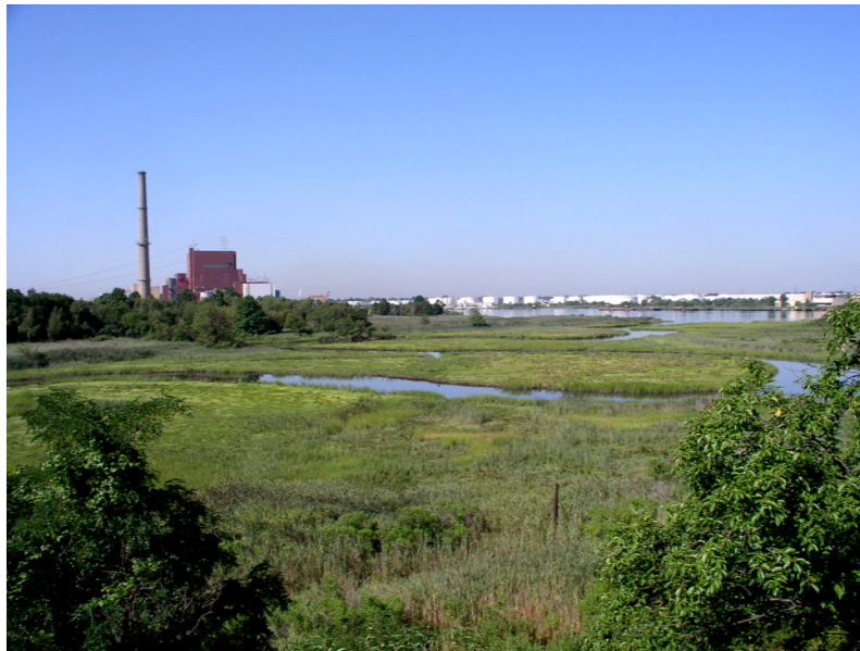
The Saw Mill Creek. Photo Courtesy Rich Shaw, NRCS
