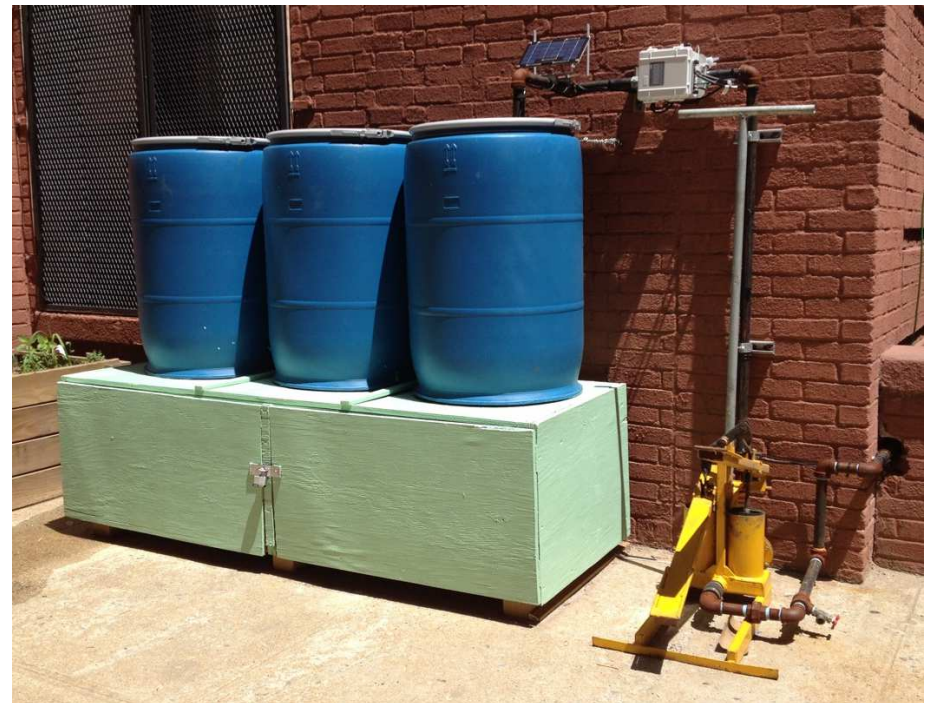
Above: A large planter was constructed in the middle of the courtyard. The floor drain is connected to a subsurface cistern in the lower courtyard. Below: The water in the subsurface cistern can be pumped to rain barrels via a treadle pump. Above the pump is monitoring data logger, which sends data via internet for remote access.
