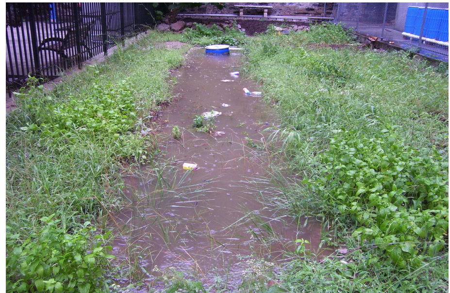
Above: The barrel in the middle is a sump that controls the flow of rainwater from the rain barrels outside the fence. Below: Despite the poor condition of the soil at the site, many of the native species, like the Spotted Beebalm in this photograph, are thriving. Weeding has been important in ensuring the natives species' establishment.
